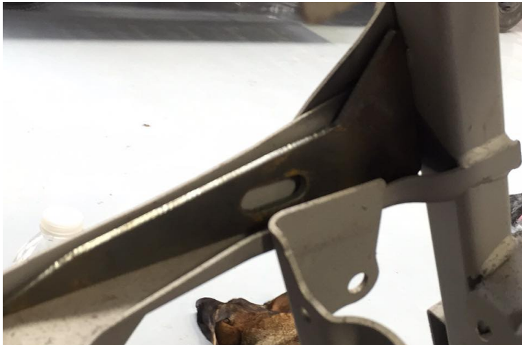
Gusset #4 inside frame between dps unit.
